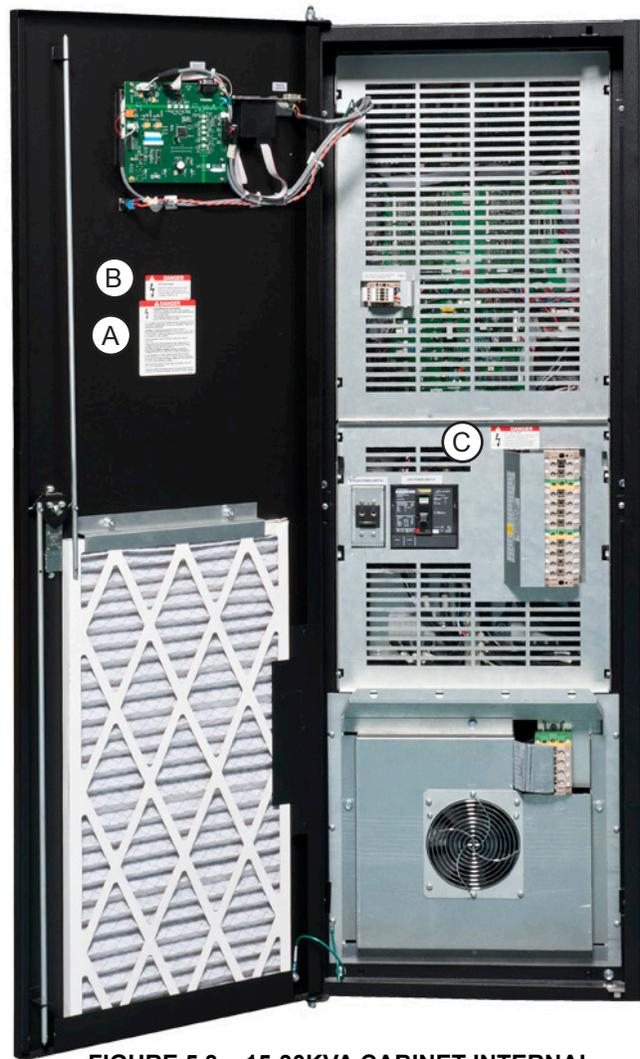
**FIGURE 5.3 – 15-30KVA CABINET INTERNAL WARNING LABEL LOCATIONS**
